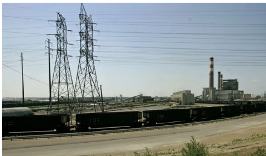
A coal power plant in Denver, Colorado, operated by Xcel Energy. (PA)
